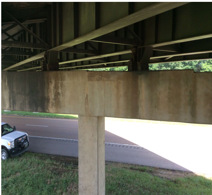
PHOTO 3 Description CRACKING AT BT 5 CAP PHOTO AT BM 3
