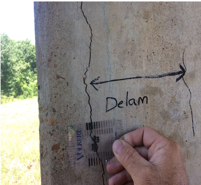
PHOTO 4 Description BT 2 column 1 delam cracks
