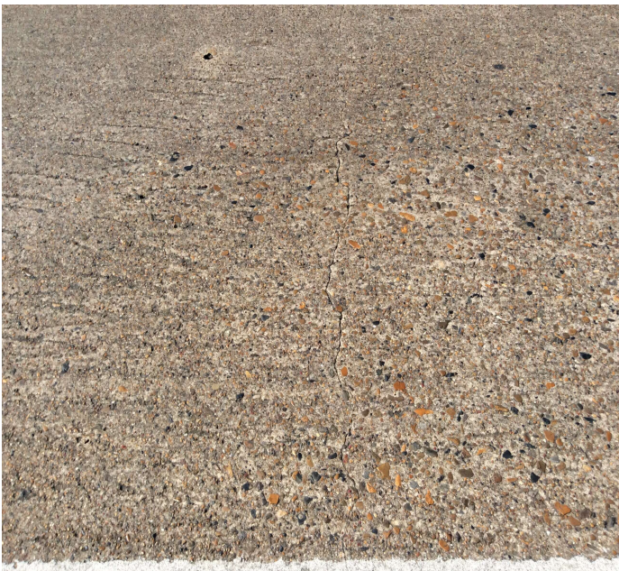
PHOTO 1 Description Sealable deck cracks all spans
