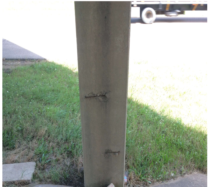
PHOTO 2 Description BT 5 spall rebar exposed ,small delam
