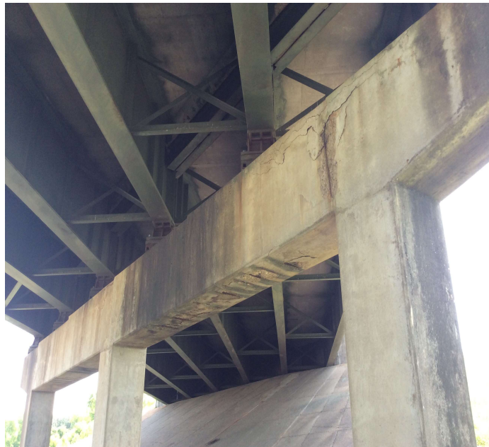
PHOTO 1 Description BT 5 DELAM, SPALL, REBAR EXPOSED
