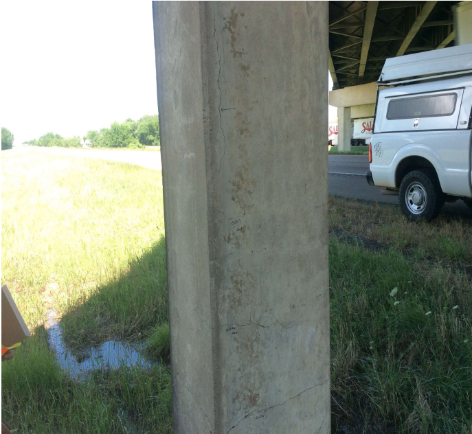
PHOTO 3 Description BT 2 column 1 horz crack.
